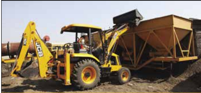
Hopper feeding for ready mix concrete
