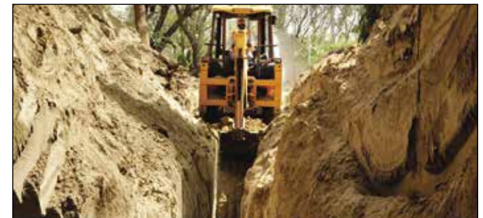
Trenching & pipe laying
