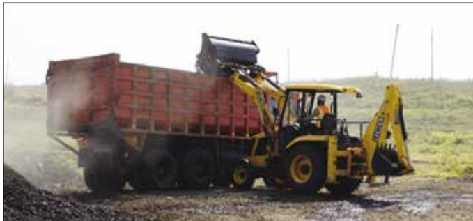
High dumper (hywa) loading
