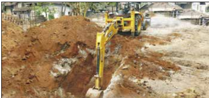
Rural infrastructure & square hole
