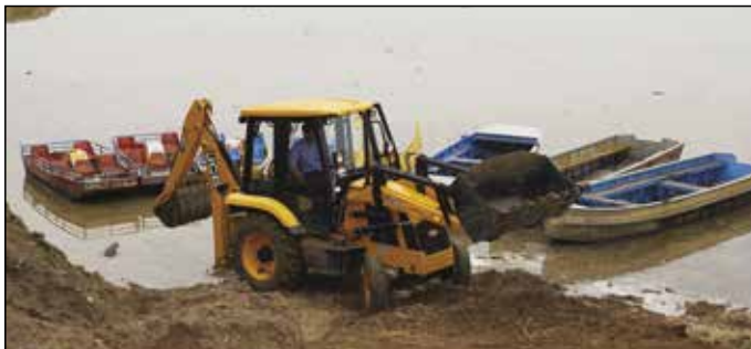
Cleaning of sewages
